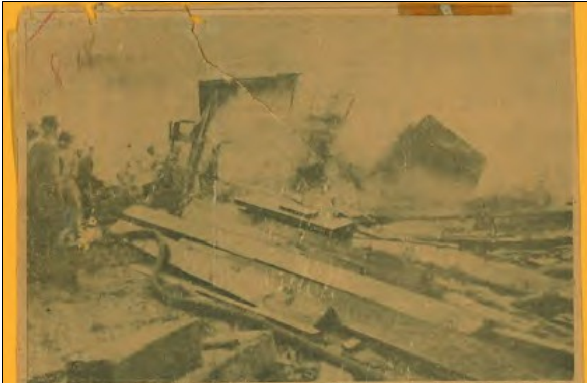
GOING, GOING, GONE —An old blacksmith shop by the Sequim Lumber and Supply Co. mill collapses as Sequim firemen pour water on the blaze, started during a high southeasterly wind last Thursday. Smoke rises from the blackened building which was a total loss. Sparks from the waste burner started the blaze. The blacksmith shop collapsed 10 minutes after the firemen arrived.
